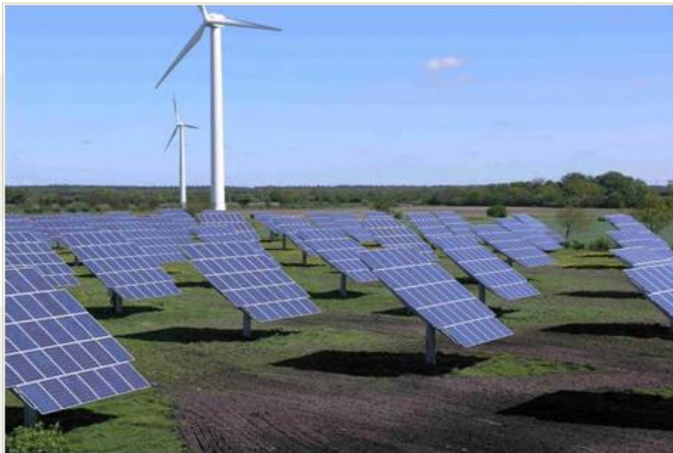
Best Practice II. – Ground PV Systems
